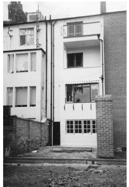
Restored rear elevation 78 Derngate
